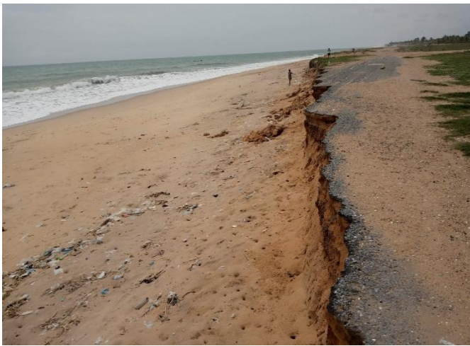
AGBODRAFO (HOT SPOT EROSION)
